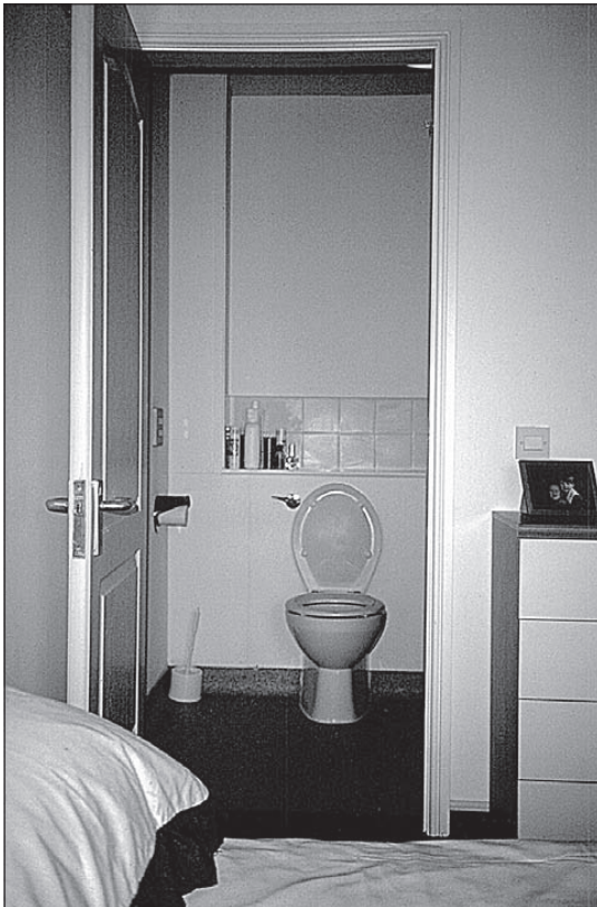
Photograph 6: WC in view from the bed with 180° door hinges and secondary low intensity lighting in en suite
